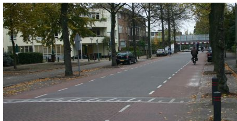
Carriageway narrowed by cycle lanes with different colour surfacing
