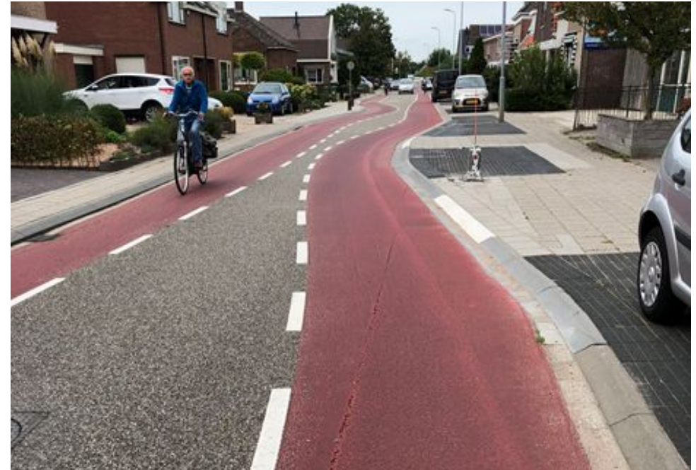
Constant width cycle lanes, in a reprofied street - Holland
