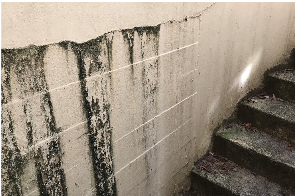
Photo 34 – Dampness to external basement access staircase wall.
