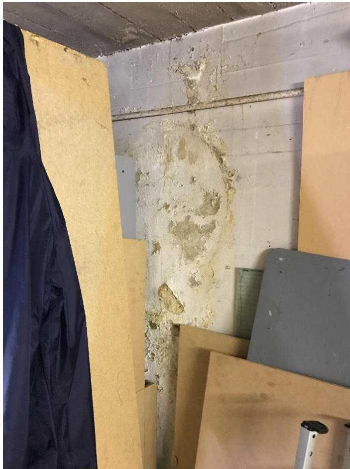
Photo 33 – Dampness to internal basement wall.
