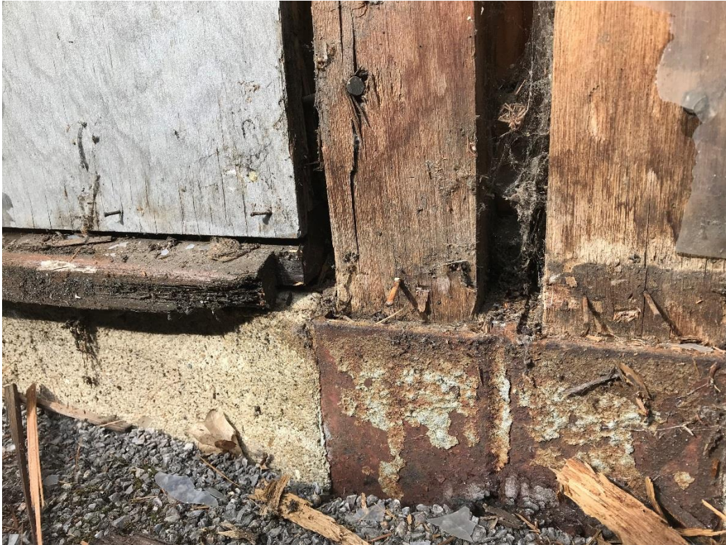
Photo 43 – Modular building, corner post base and shoes.
