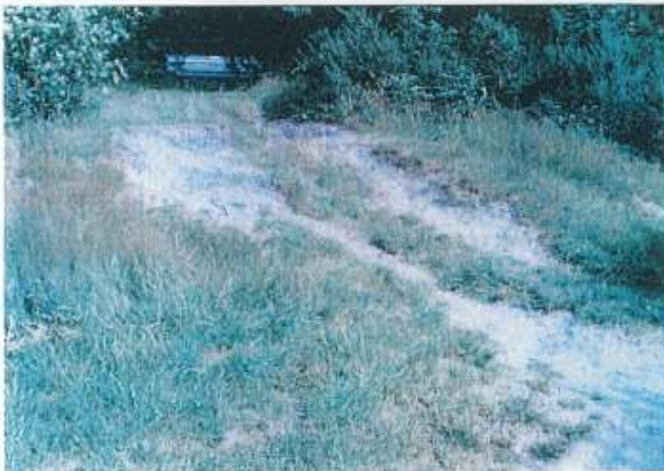
Plate 7 – Evidence of intense runoff erosion feature feeding directly into the lake
