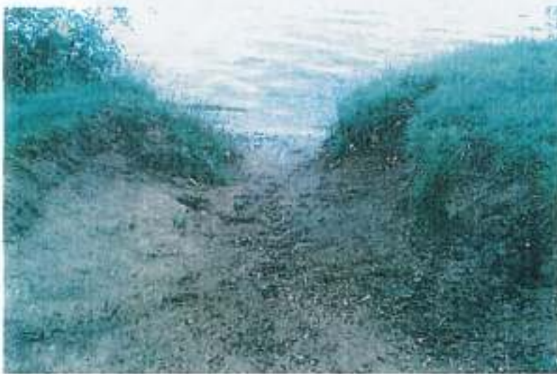
Plate 4 – Lack of defences has led to erosional features in the margins
