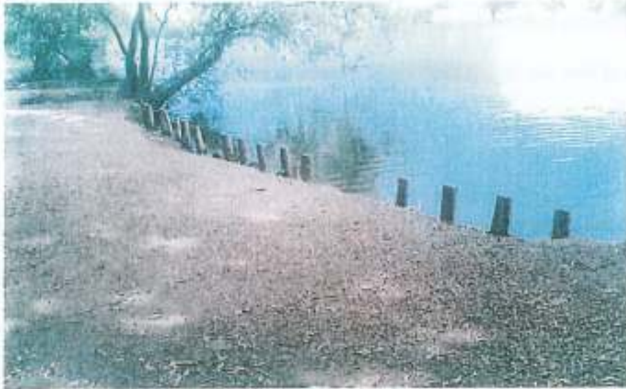
Plate 2 – Existing erosion control measures employed at certain points around Petersfield Heath Lake.
